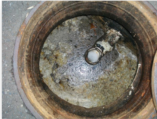
Figure 3: Contaminated Grease Trap
