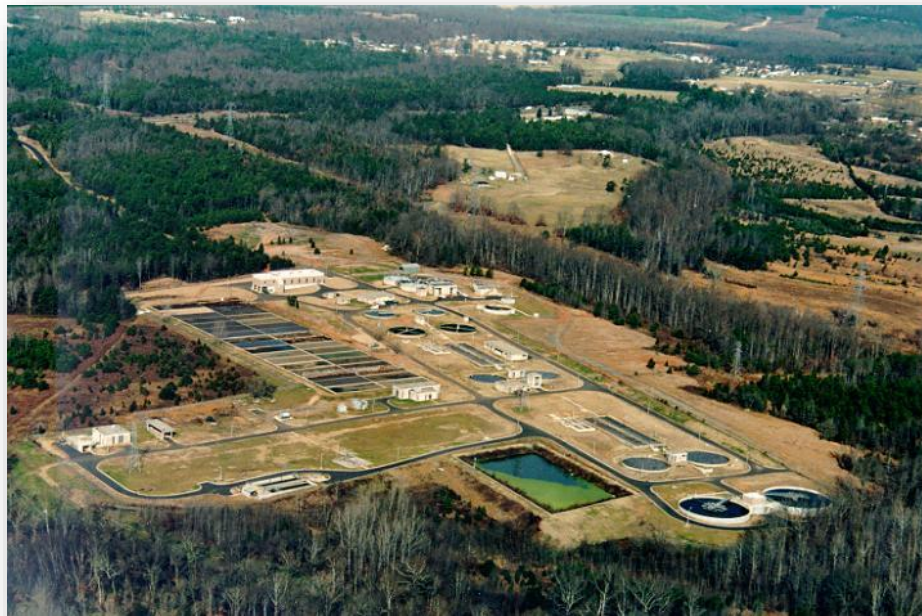
Figure 2: Mallard Creek Water Reclamation Facility
