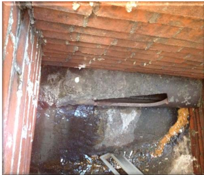
Figure 5 – Broken 8-inch Sewer Mainline in Storm Catch Basin
