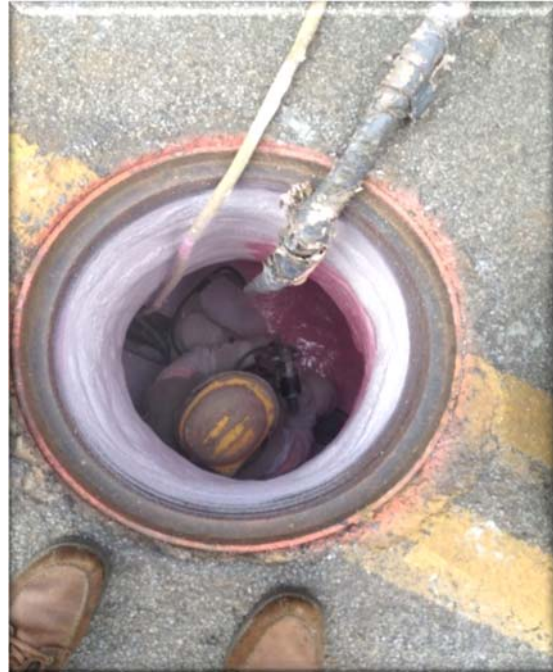
Figure 12 – Manhole Rehabilitation
