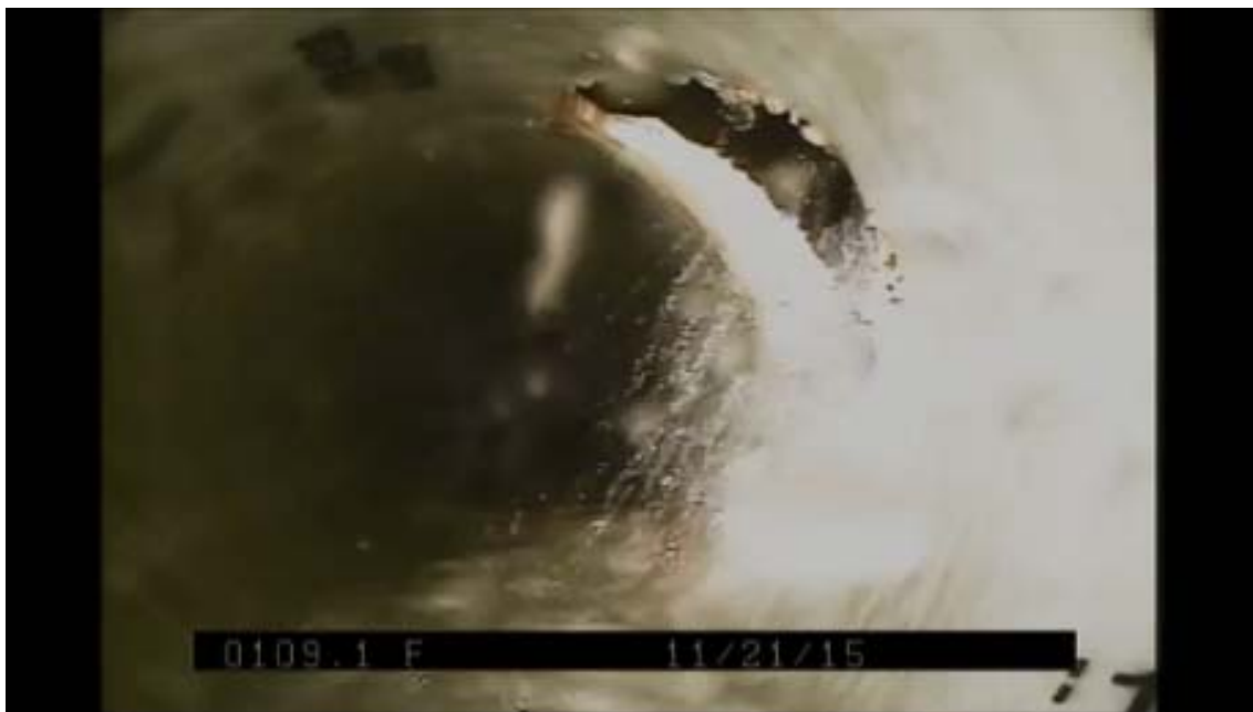
Figure 21 – Leaking Service Connection – Core & Brushed Only
