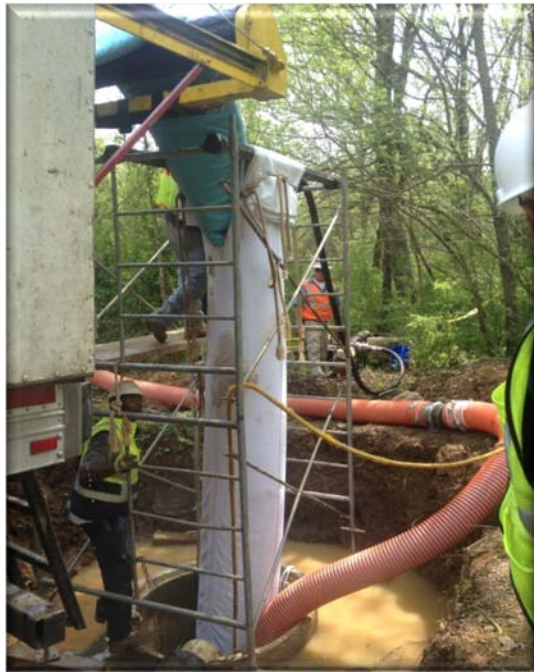
Figure 11 – CIPP Mainline Repair
