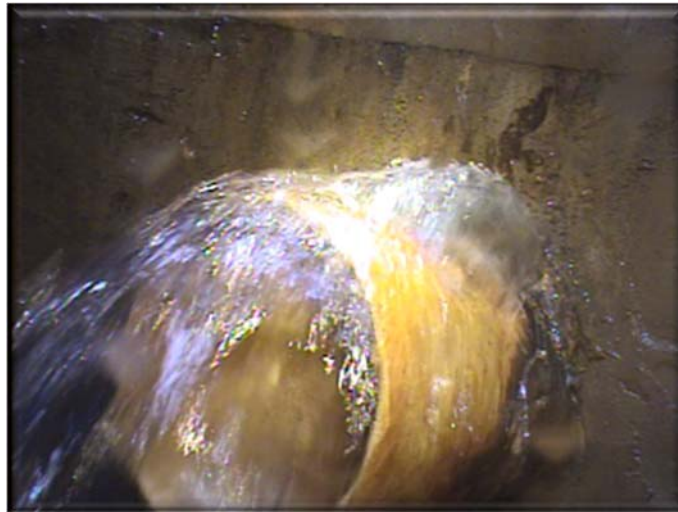
Figure 6 – Active Infiltration at Manhole/Line Connection
