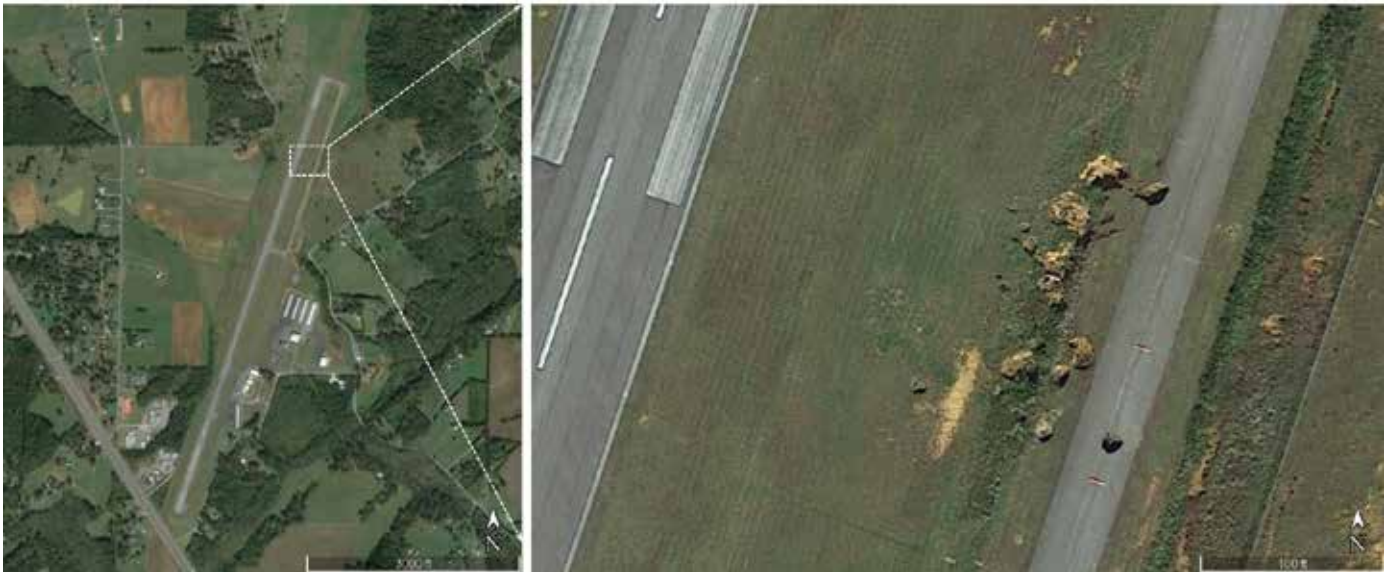
Figure 1: Sinkholes adjacent to taxiway (Google Earth Pro images dated 10/14/2015).
