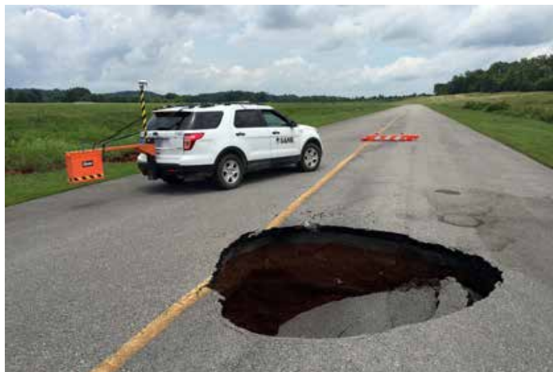
Figure 10: Photo of GPR system adjacent to sinkhole in taxiway (view to the north).
