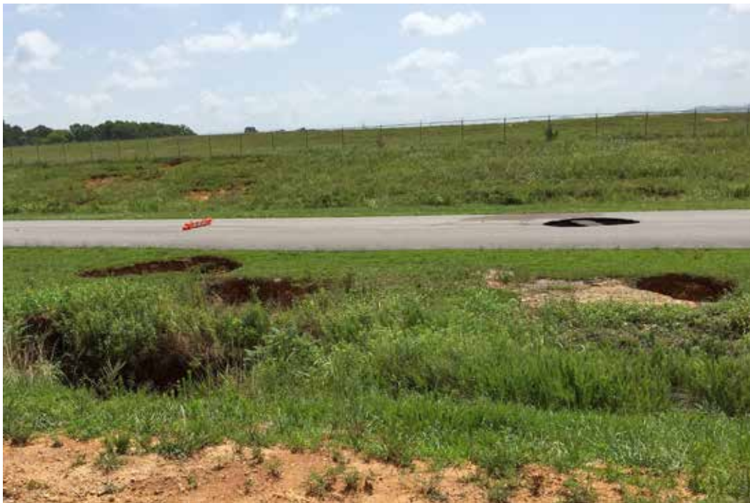
Figure 2: Sinkholes adjacent to and within taxiway (view to the east).
