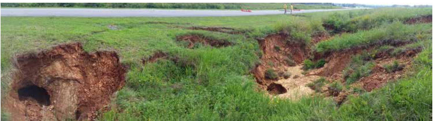
Figure 3: Sinkholes adjacent to taxiway along drainage ditch (view to the south).
