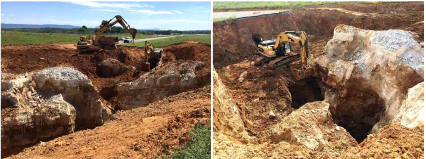
Figure 7: Irregular/pinnacled bedrock exposed within the area of the sinkhole cluster during the current remediation portion of the project (view to the south).
