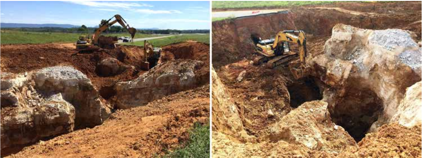
Figure 7: Irregular/pinnated bedrock exposed within the area of the sinkhole cluster during the current remediation portion of the project (view to the south).
